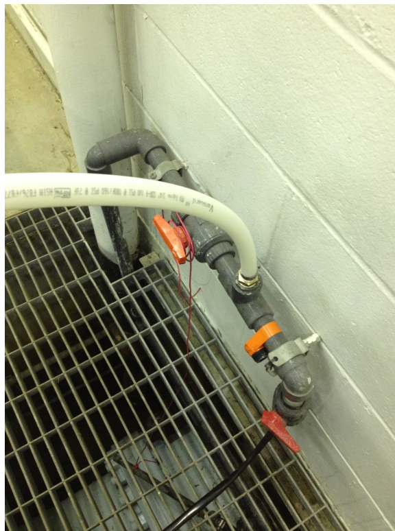
Figure 16: Brine solution injection connection.
